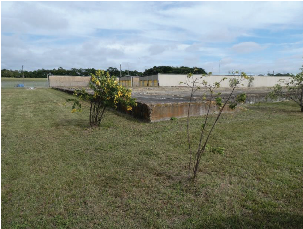
Concrete slab on site with off-site storage units in background
