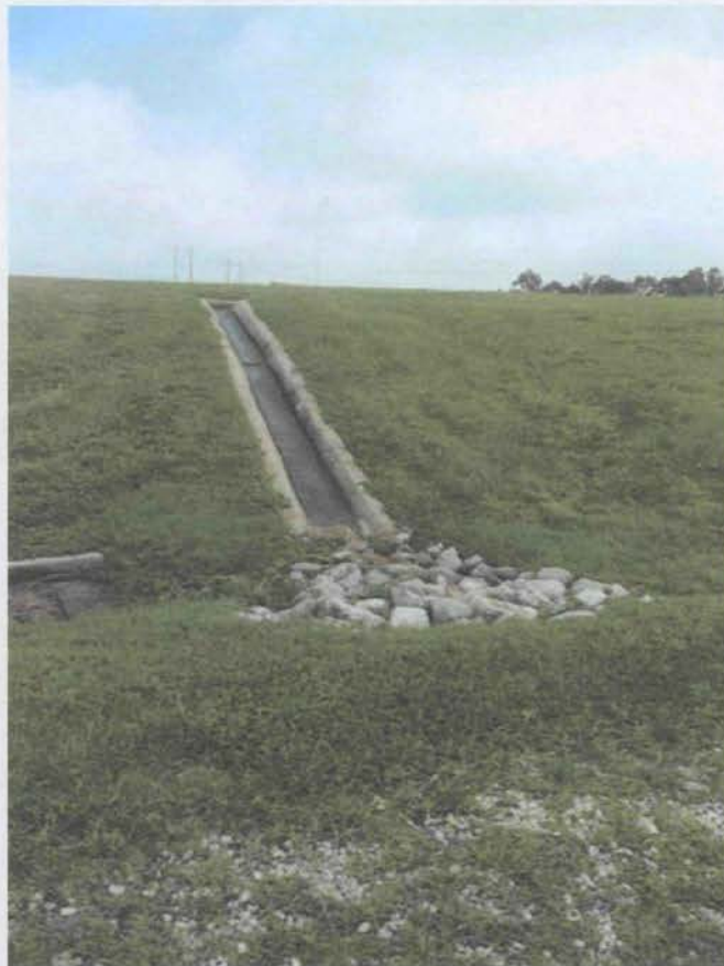
Water drainage area to prevent erosion of the RCRA cap.
